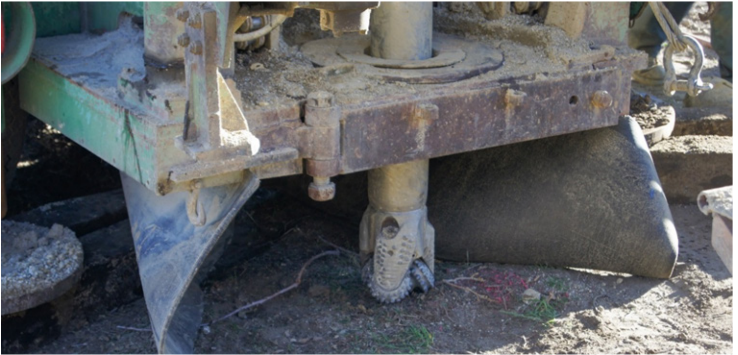
7-inch drill bit was used to drill borehole in project.
