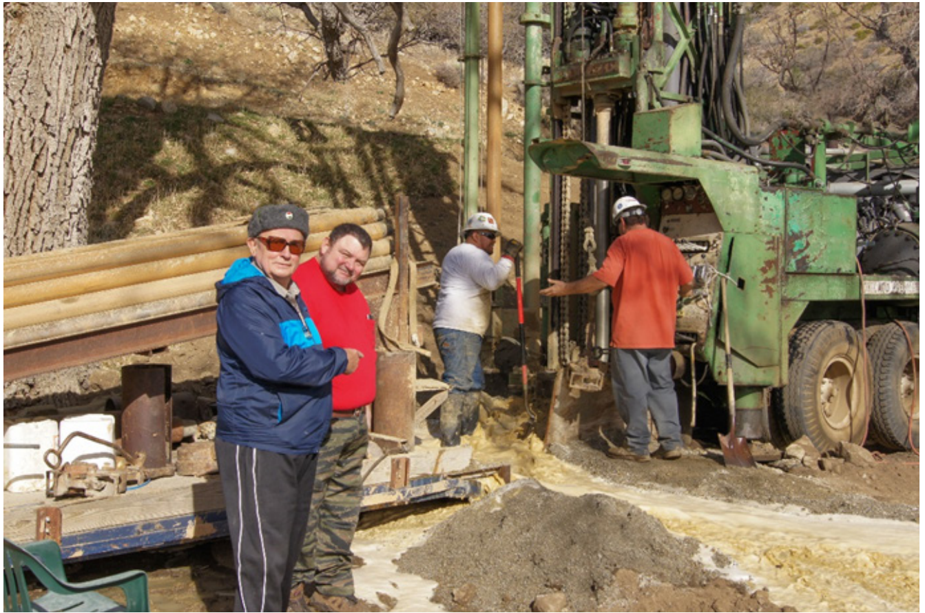
Pal and Ben with the drillers. Water and debris encountered at 50 feet at final phases of drilling.
