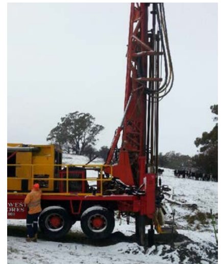
Australian DSW Drilling Project for farmer
